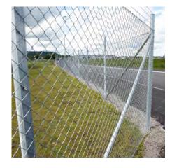
Produced out of steel wire in Magnelis or PVC coated galvanized wire
